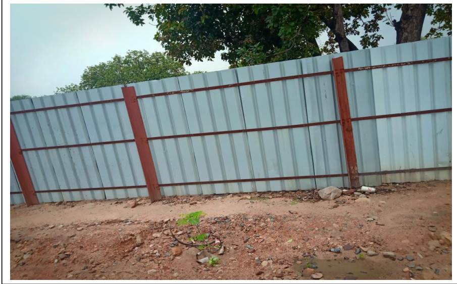
View of Wind Braking Wall
