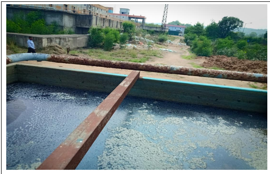
Non operational Sewage Treatment Plant (Compact)
